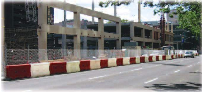
The TrafFix Water-Wall used as a Longitudinal Barricade along a job site.
